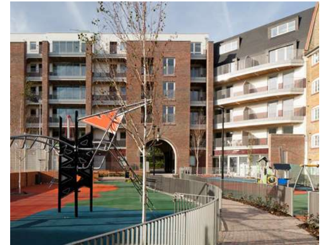
Estate regeneration including new mixed tenure homes, a community centre and a Multi-Use Games Area for social and physical well-being. Bourne Estate, Holborn, London.
